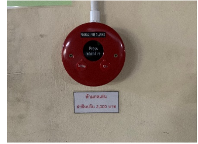
fire alarm manual station
